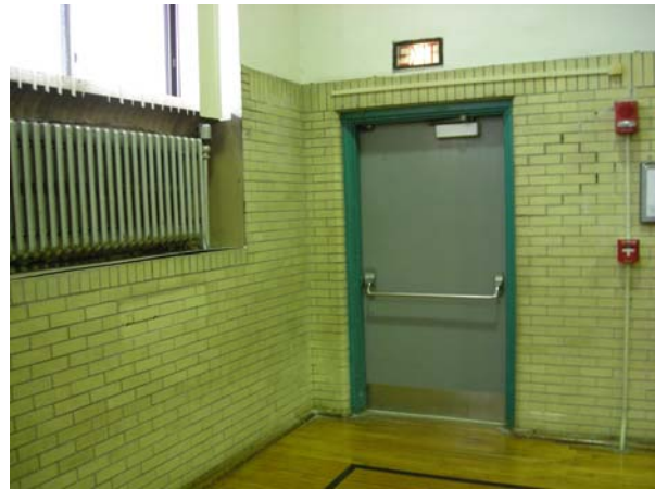
Radiator in Gymnasium
