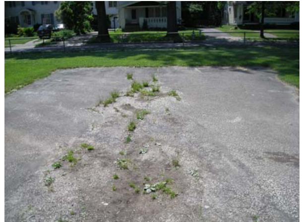
Deteriorated Playground Asphalt
