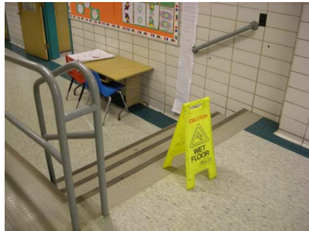
Stair and Ramp
