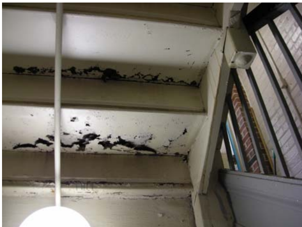
Peeling and Corrosion on Underside of Stair
