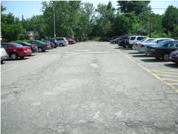
Deteriorated Asphalt in Parking Lot
