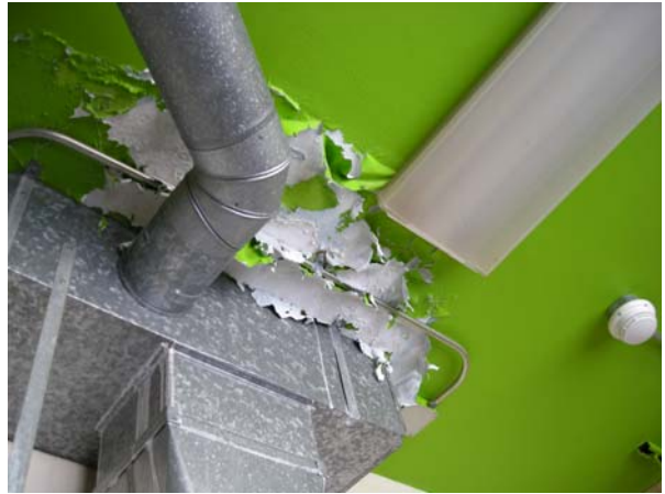
Ceiling Deterioration
