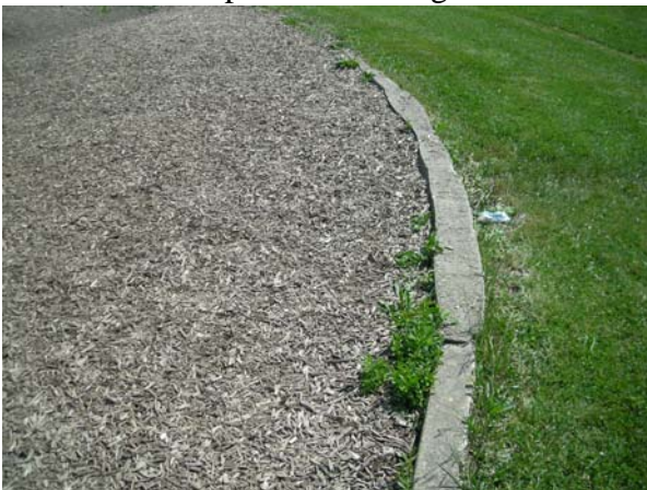
Concrete Playground Curb
